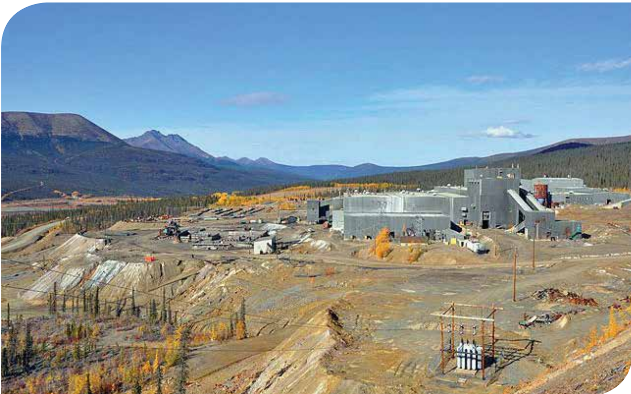
Derelict Faro Mine closed in 1998 was once one of the world's largest zinc mines. Photo Credit : Yukon News
